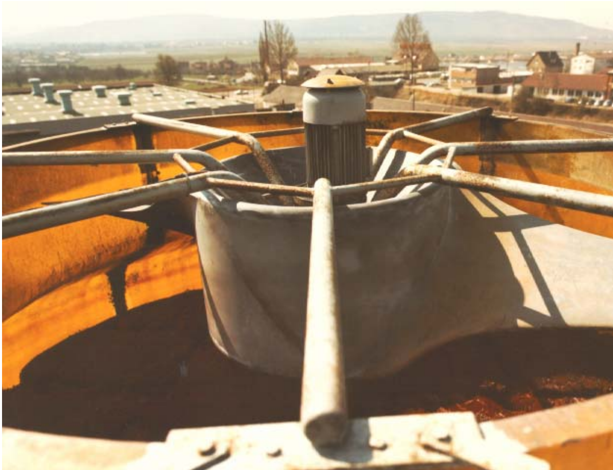
Fig. 29 Geared motor in V1 mounting driving a cooling tower fan Fan impeller diameter up to 3.4 m Typical factors of inertia FI up to 30
