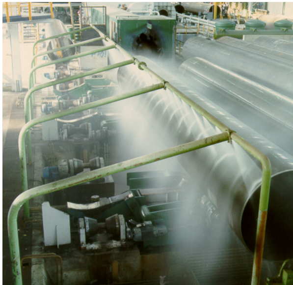
Fig. 4.4.4 Descaling large pipes using a high-pressure water jet Roller table motors and auxiliary drives to degree of protection IP66
